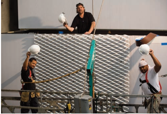
Workers begin installing building's mesh cladding
